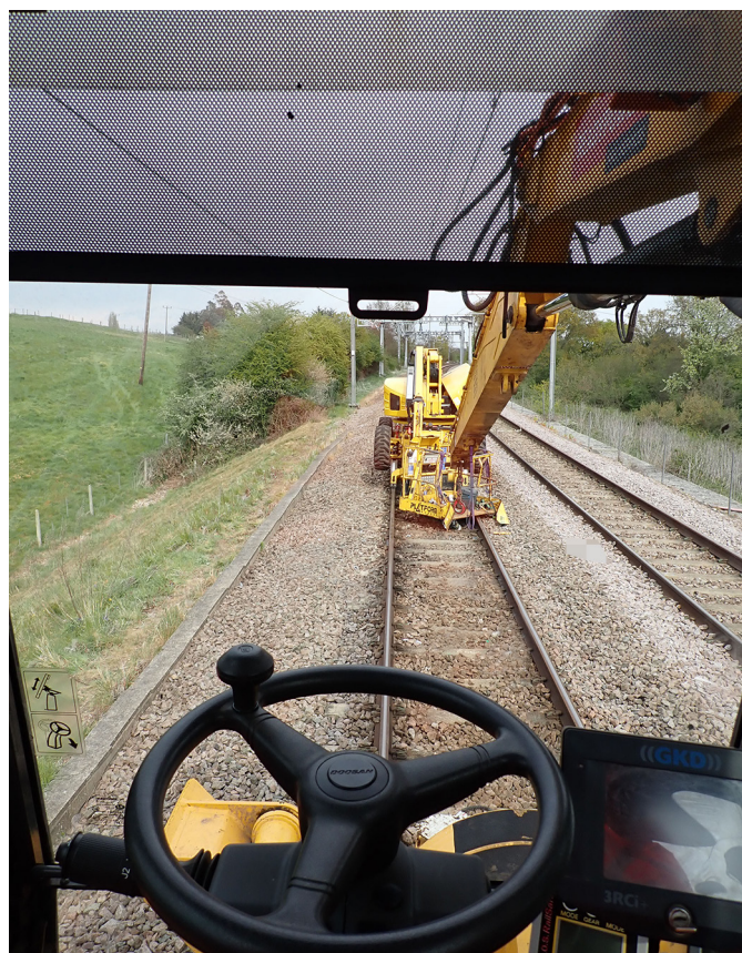
Figure 7: The view from the crane operator's seat with the sunshade drawn at the accident location (in daylight)
