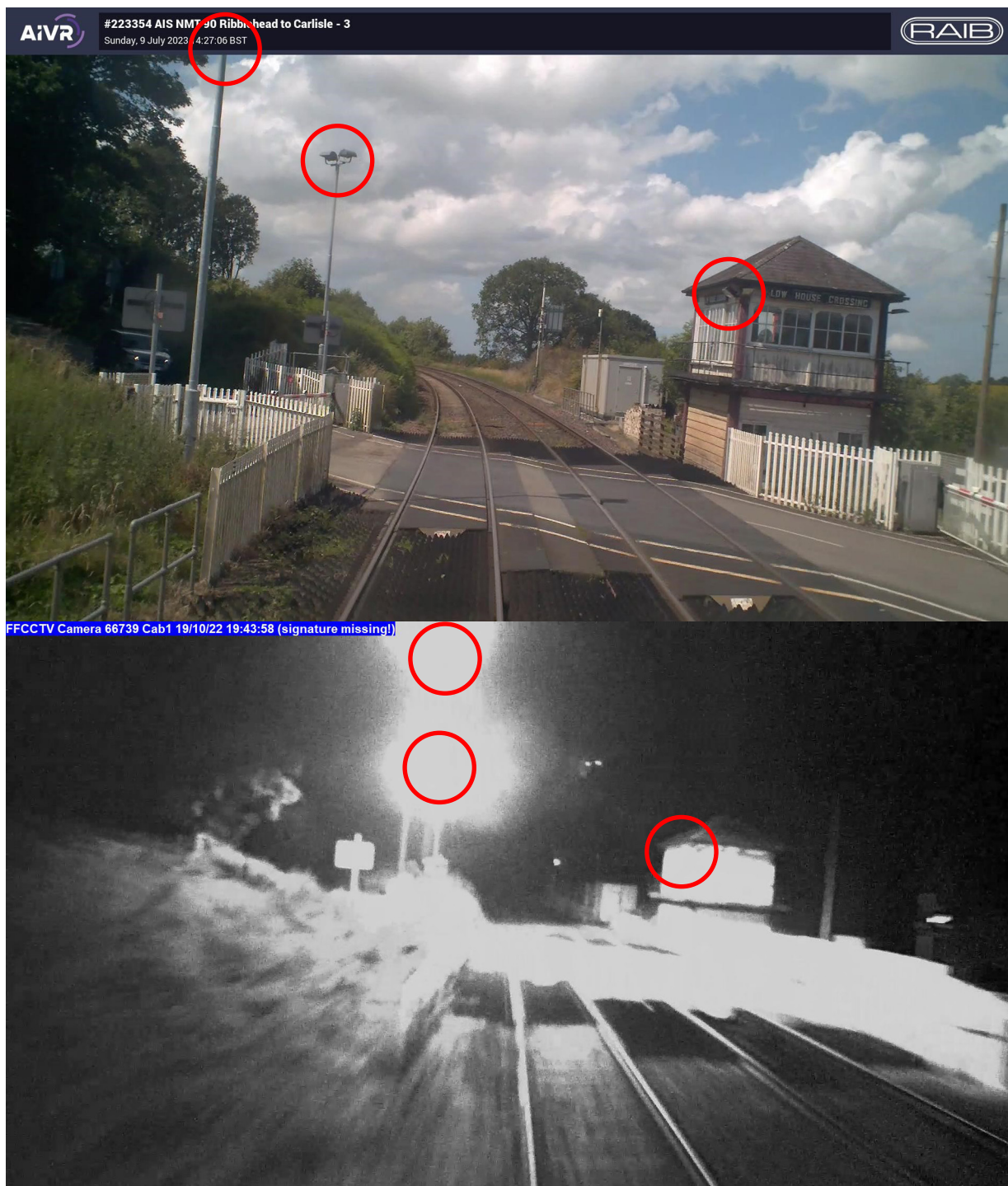
Figure 39: Low House signal box, with floodlights circled (top image courtesy of Network Rail, bottom image courtesy of GB Railfreight).
