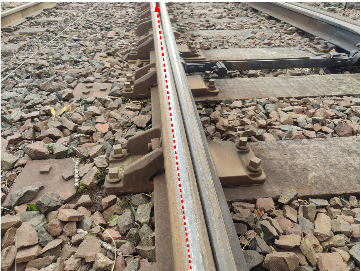
Figure 30: False flange marks at Kirkby Stephen.
