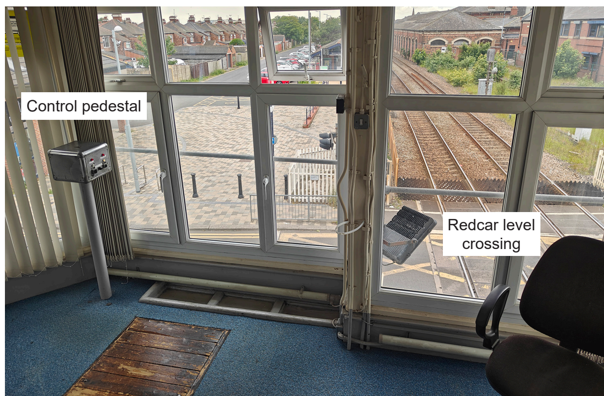
Figure 6: Redcar level crossing and control pedestal.
